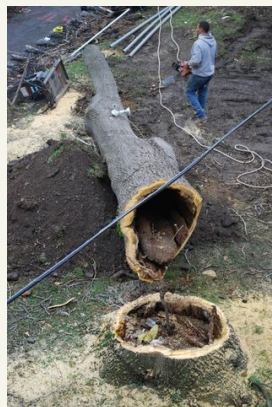
Pictures from Backyard Project (Left to Right) The foundation to the new gazebo area, The old Apple Pi Tree, and the new foundation to the basketball court
